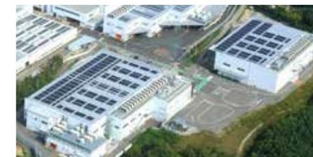
Figure 11: Nishi-Kobe Works: 927-kW power generation facility (of which 422 kW is sold via FIT)
